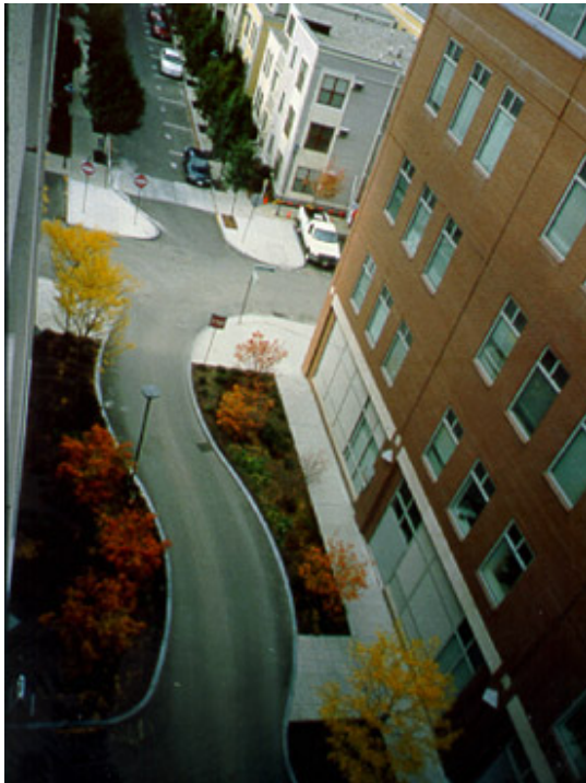
Serpentine street uses a winding pattern to slow down vehicle speeds
