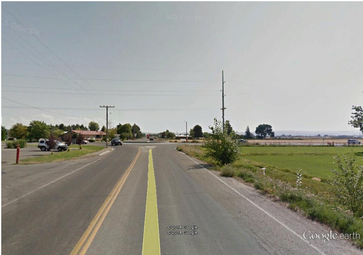
Figure 4. Iona Road Facing N 25 th E, Eastbound
