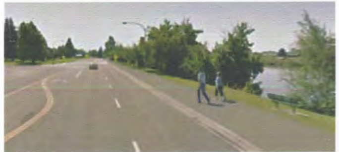
Preferred Option/Option A: Five lane intersection configuration. North of intersection, preferred option narrows to four lanes (adding a buffer traiside) and Option A remains five lanes.
