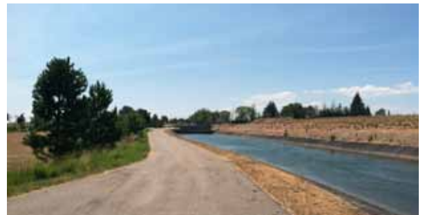
Figure 3.2. Existing canal trail on the northwest side of Snake River Landing.
