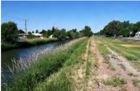
Figure 3.1. Existing canal and maintenance access road south of 14th Street.
