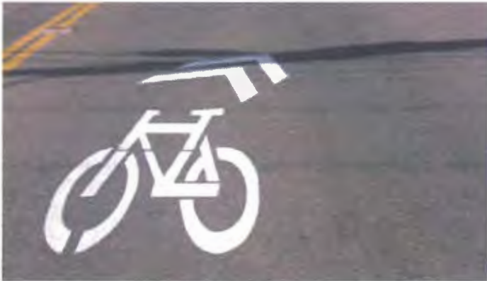
Example of wayfinding shared lane markings from Jackson Hole, WY (Project #9).
